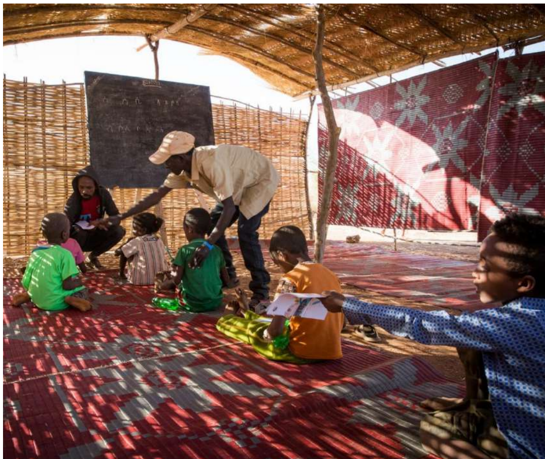
A temporary learning space in Um Rakuba Camp, Sudan. In the space of a week, the team erected school structures that can host 700 children in two shifts. The teachers are themselves refugees that can now teach again. Photo: Ingebjørg Kårstad/NRC
